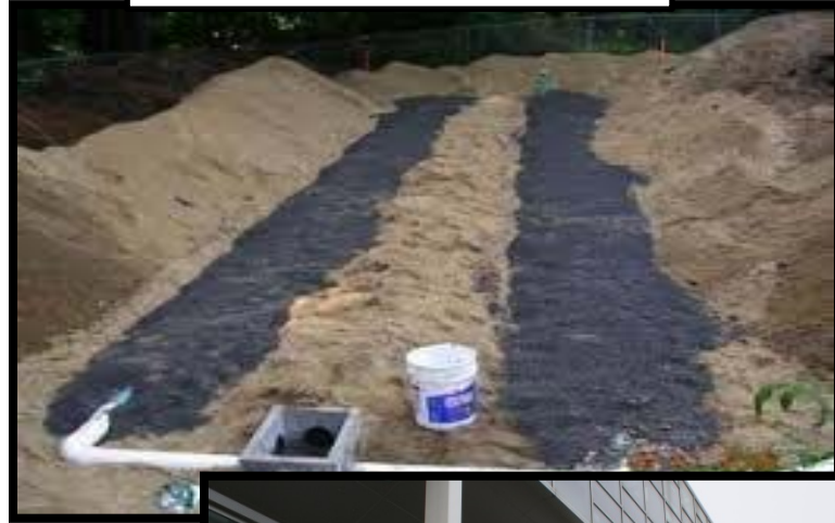
New septic system Installation
