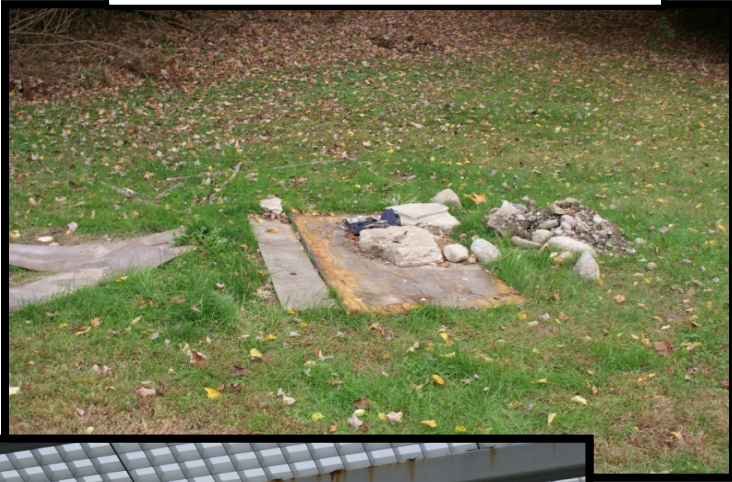
Old septic system distribution box
