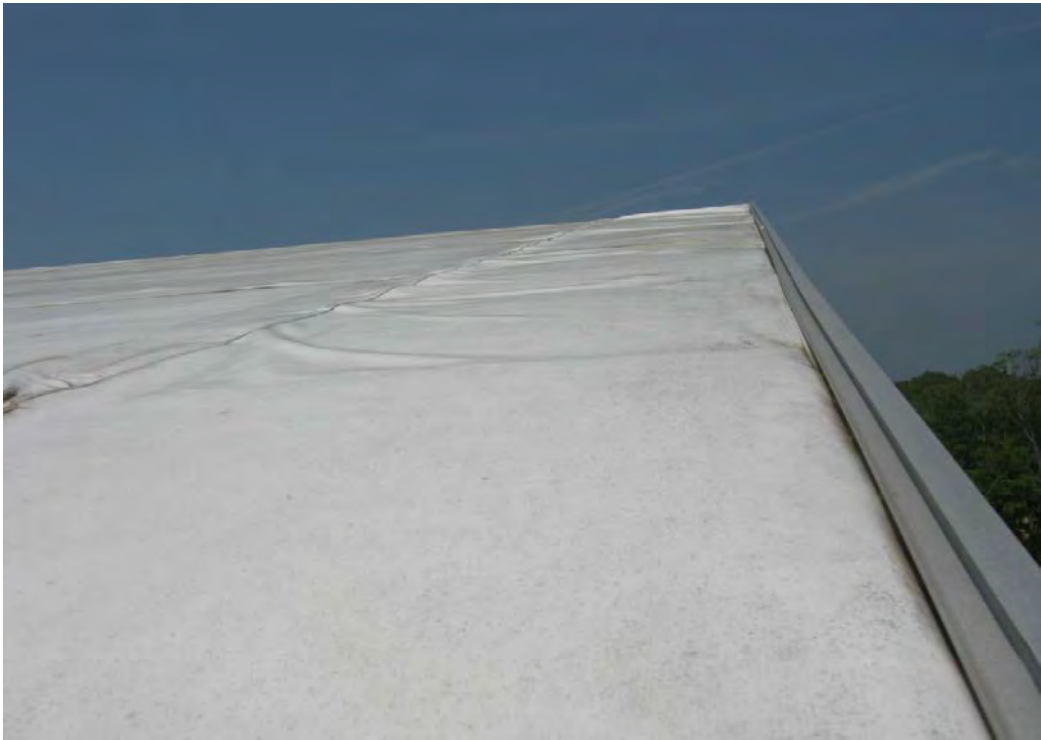
Roof membrane failures and patches around skylight
