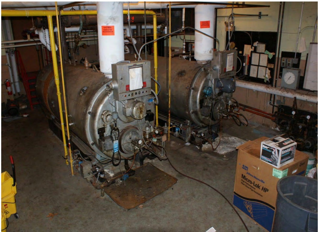
Old 1964 boilers showing age and leaks
