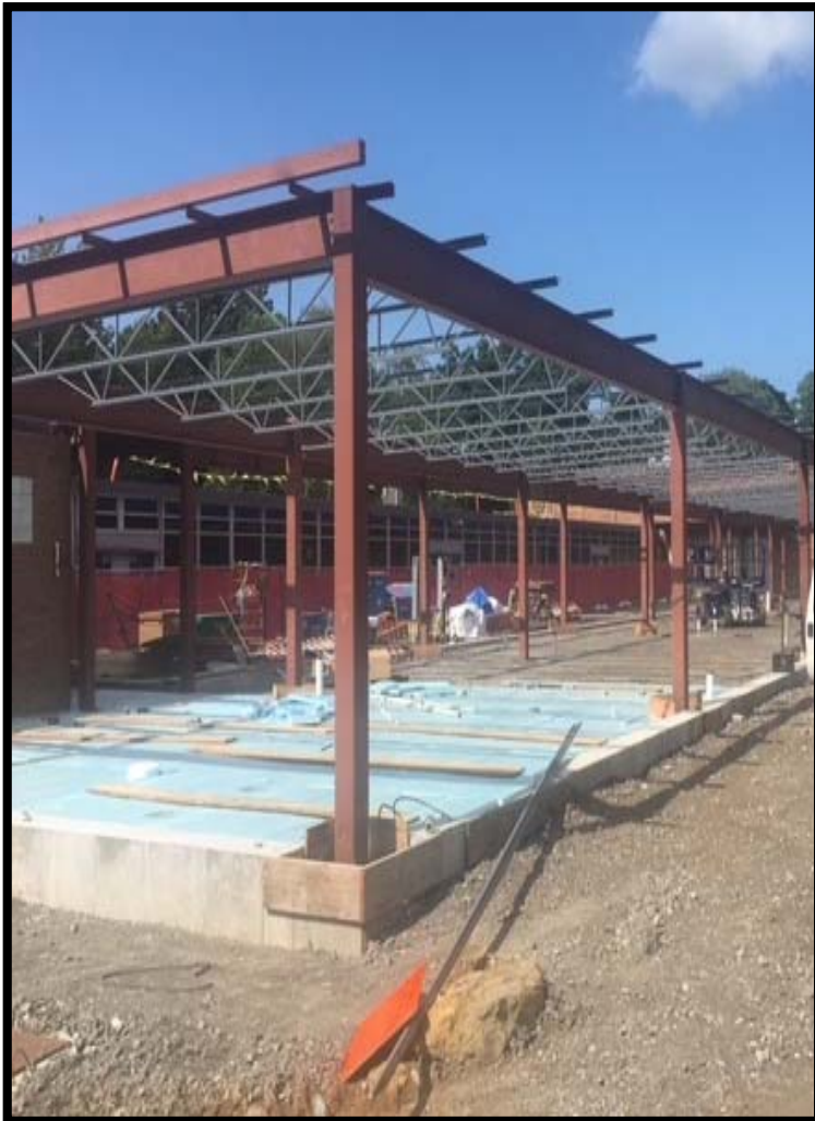
Holland Hill Elementary School Project Under Construction August 22, 2018
