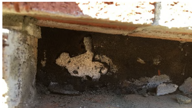
Black Vapor Barrier on CMU Block Wall (Gymnasium South Wall)
