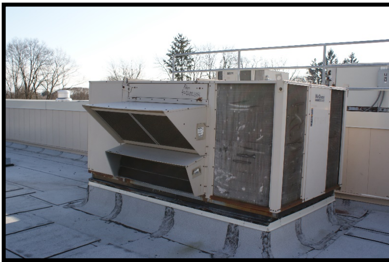
FWMS Replace Main Office HVAC RTU
