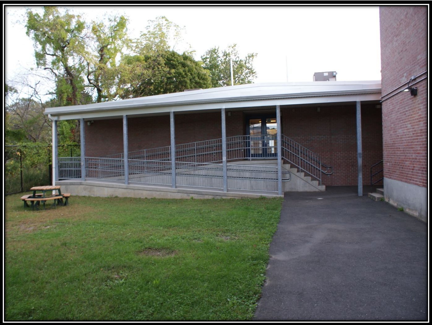
Sherman School annex building view
