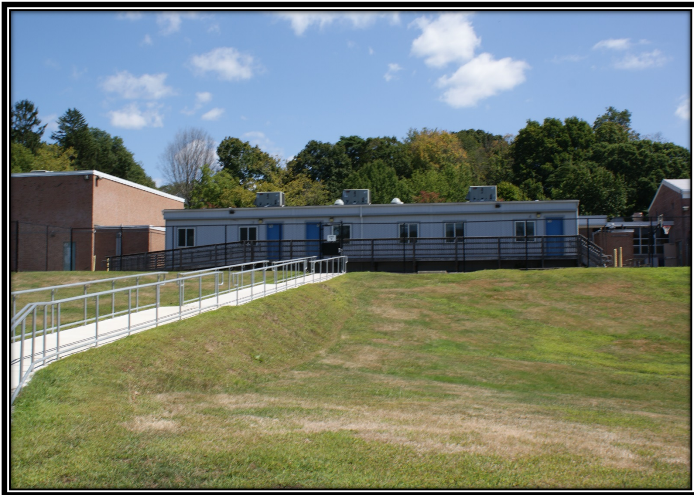
Mill Hill School portable (temporary) classrooms triple unit
