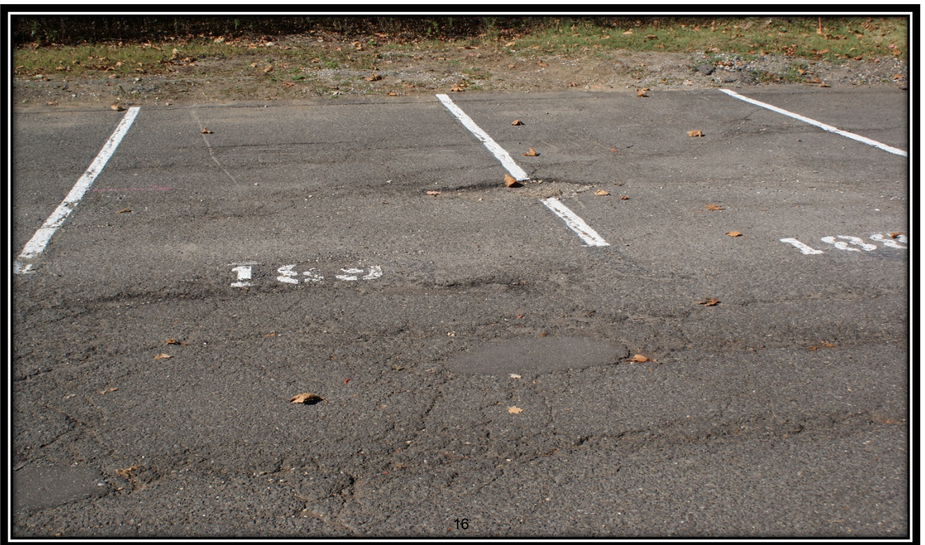
FLHS student parking lot deteriorating bituminous paving showing cracks and several patches
