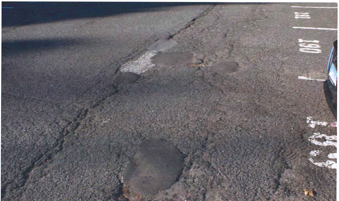
FLHS student parking lot deteriorating bituminous paving showing cracks and several patches
