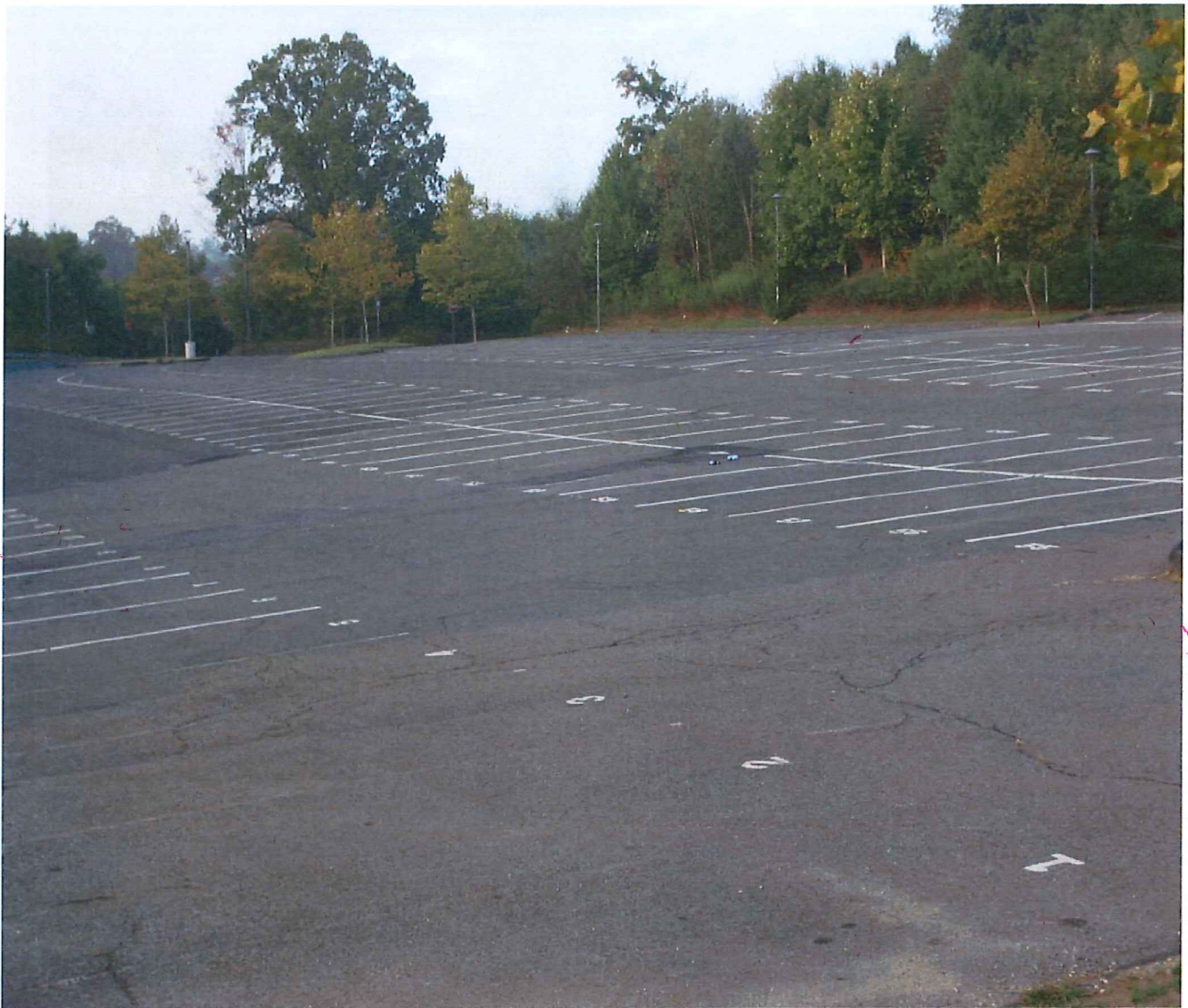
FLHS student parking lot deterioration after more than 12 years of use
