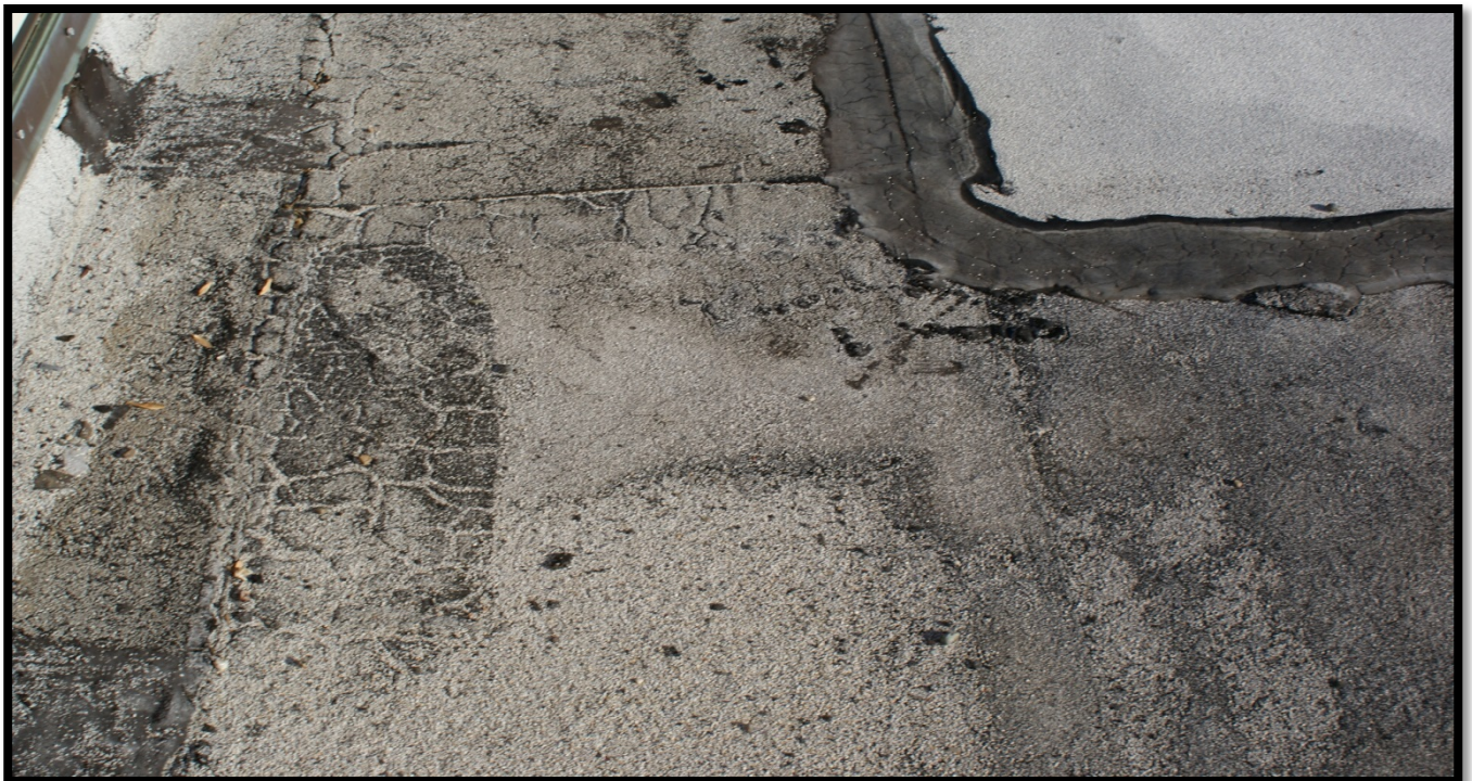
Fairfield Woods Middle School Deteriorating Roof Conditions
