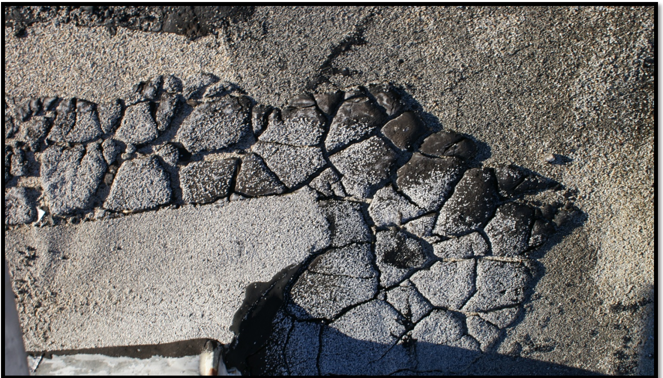
Fairfield Woods Middle School Deteriorating Roof Conditions “Close-up”
