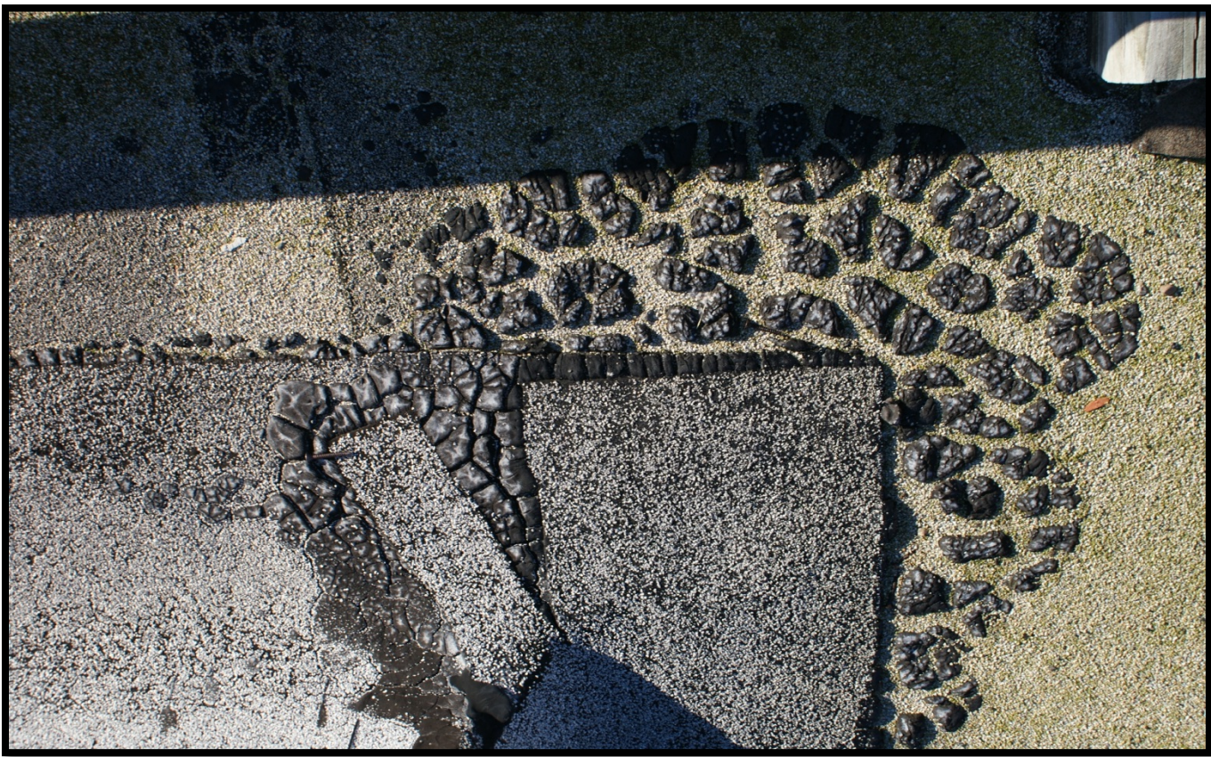
Fairfield Woods Middle School Deteriorating Roof Conditions “Close-up”
