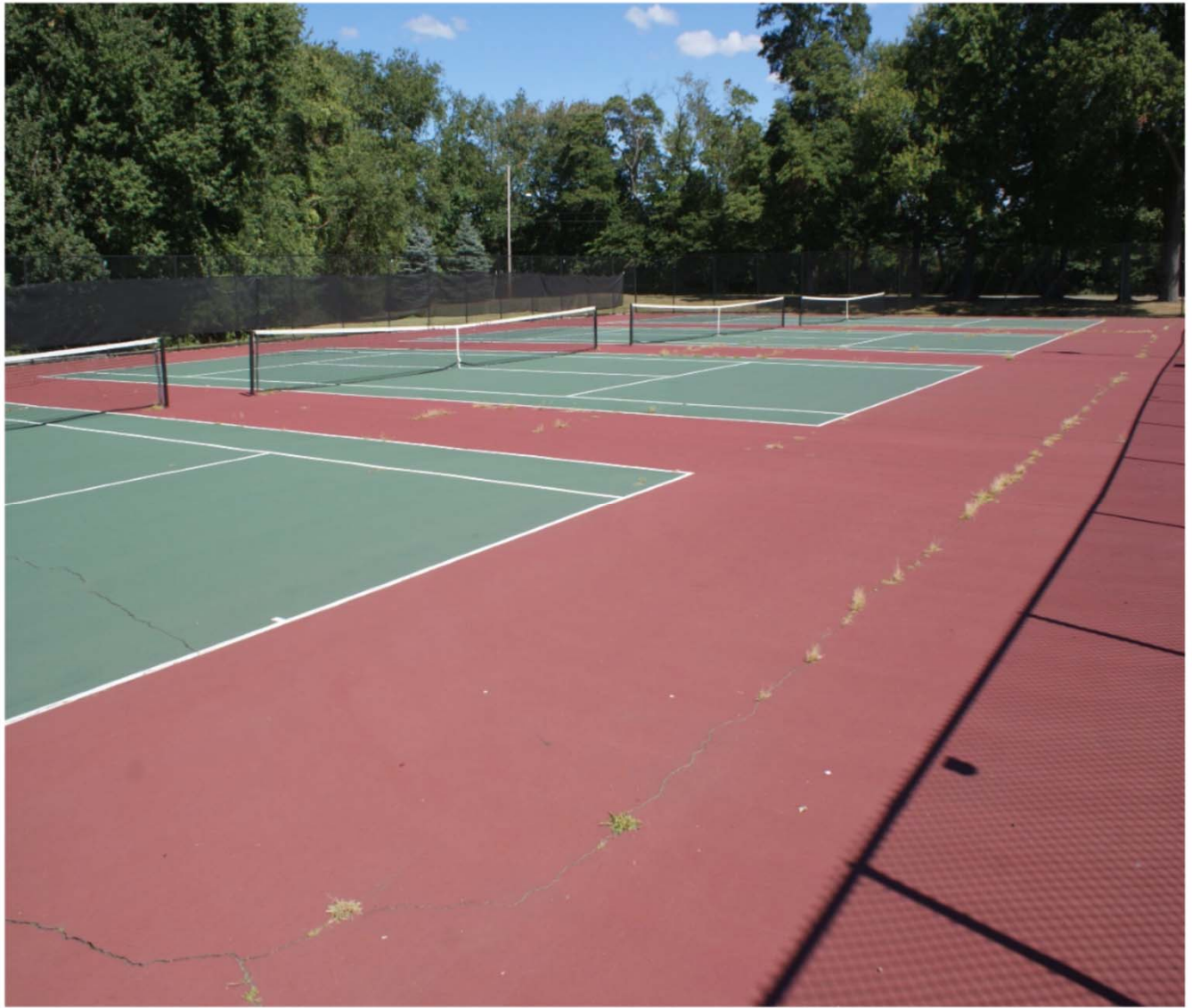
FWHS existing Blake Tennis Courts in poor deteriorating condition – unsafe for play
