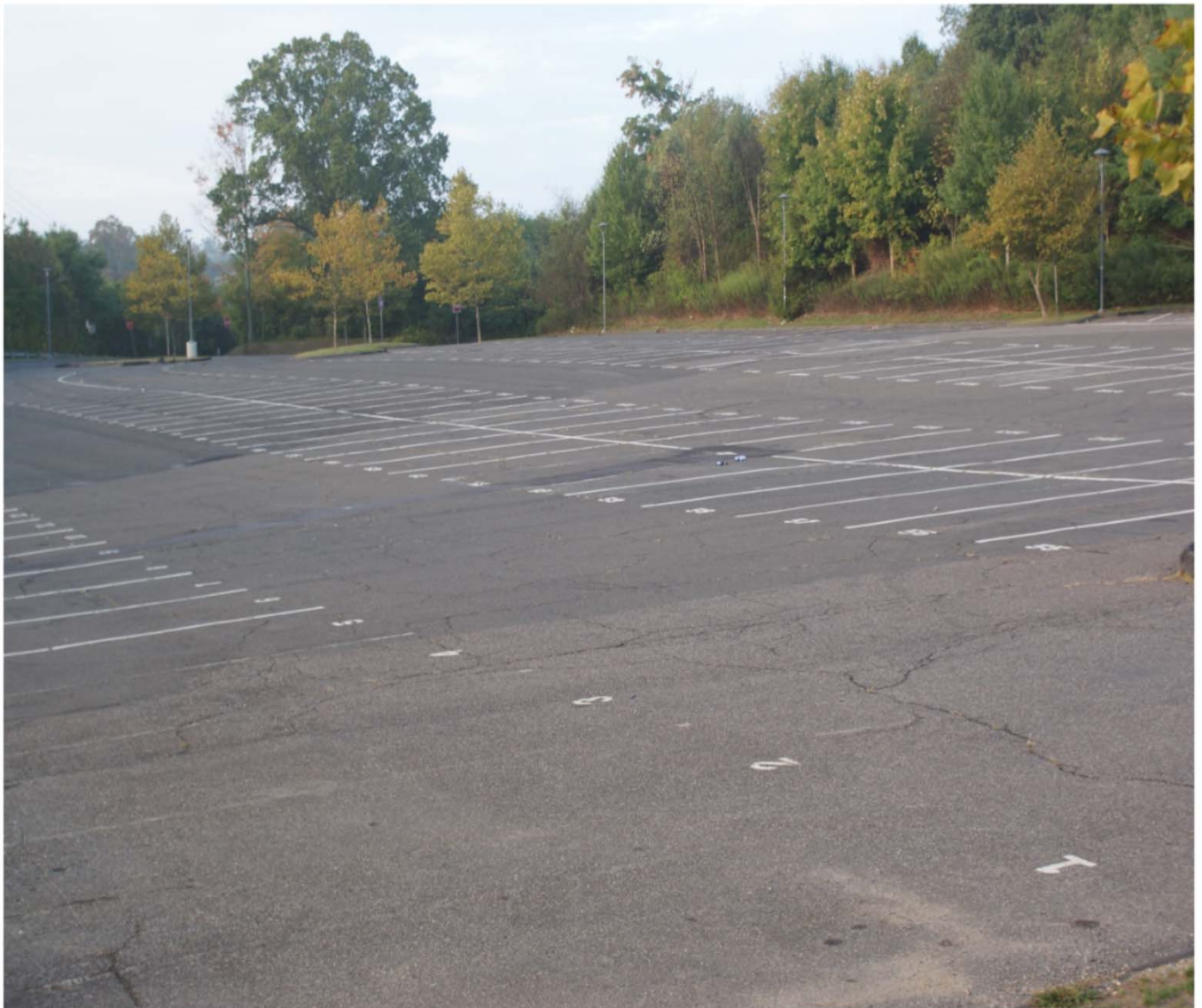
FLHS student parking lot deterioration after more than 12 years of use
