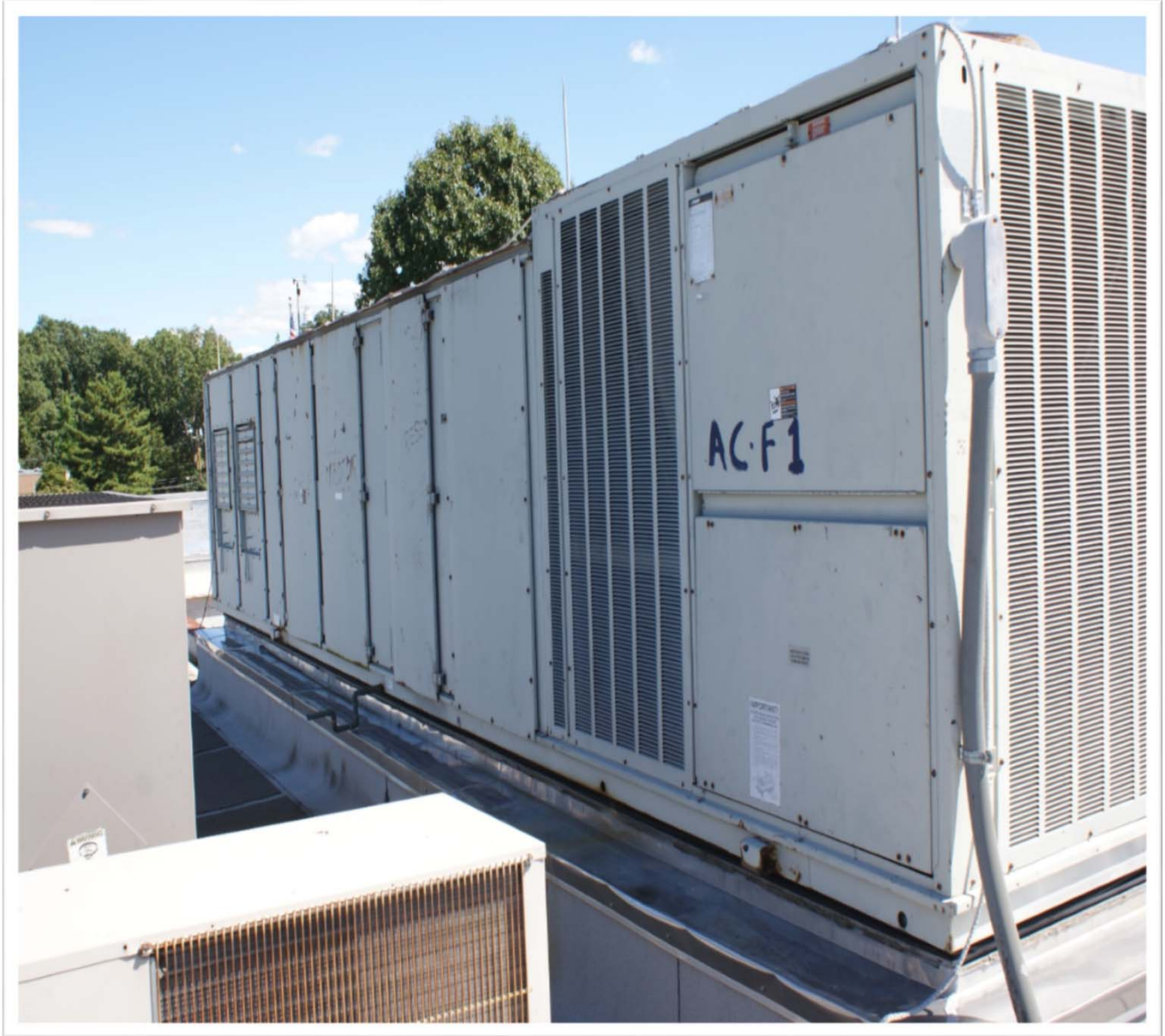
FWHS Library Media Center HVAC rooftop unit in failing deteriorating condition
