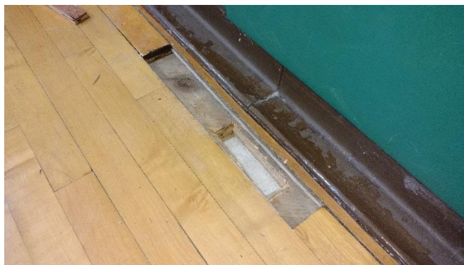
Typical Wood Flooring and Underlying Materials
