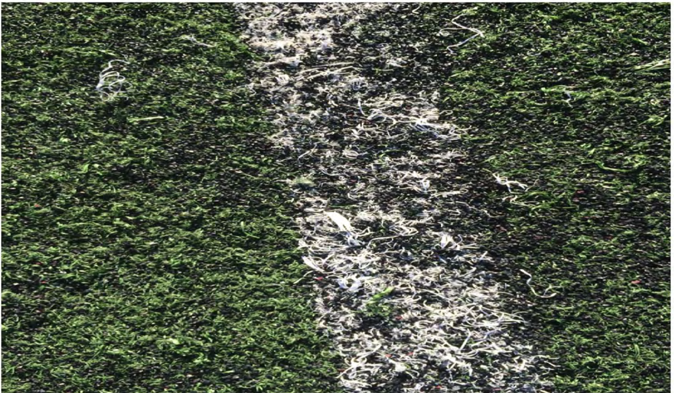
Old 2004 artificial turf field showing age and deterioration
