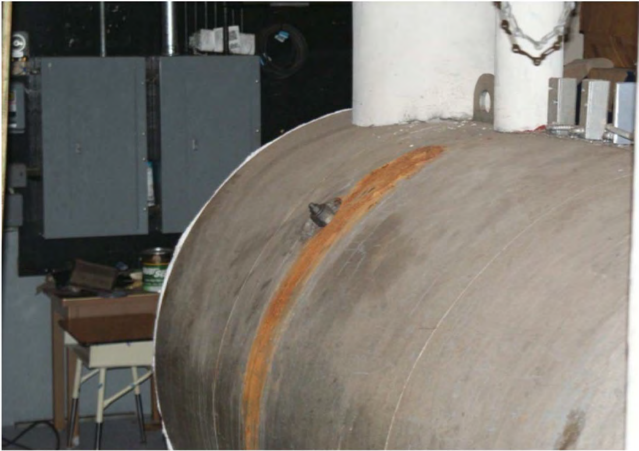
Old 1966 boilers showing age and leaks
