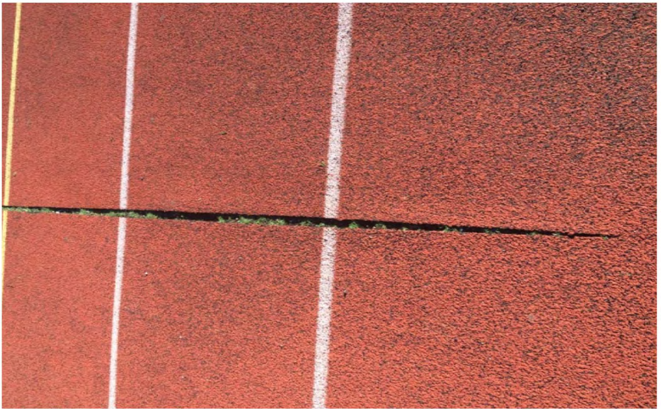
Old 2004 artificial running track showing age and deterioration
