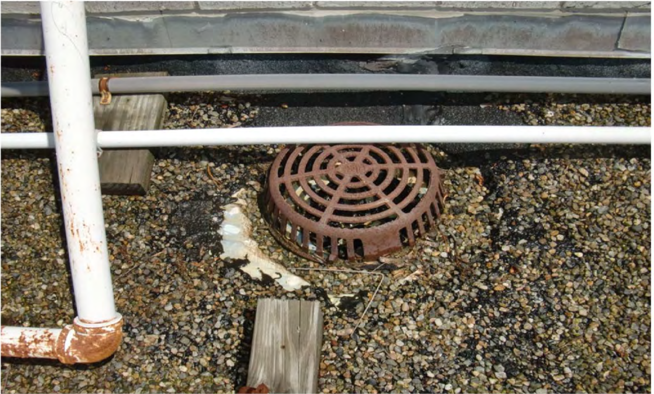
More roof patches and ponding of water failures
