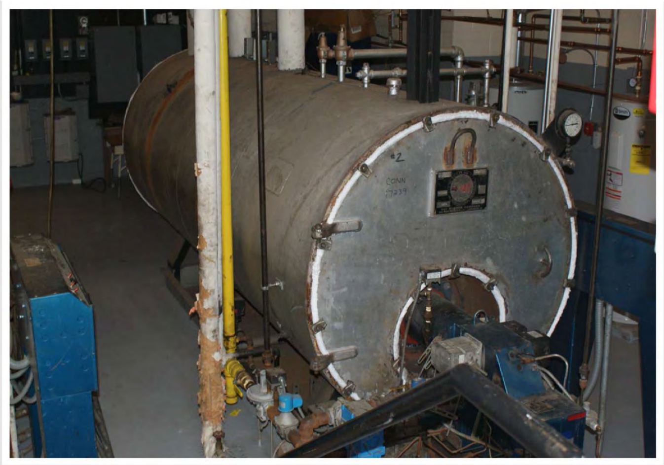
Old boiler photos
